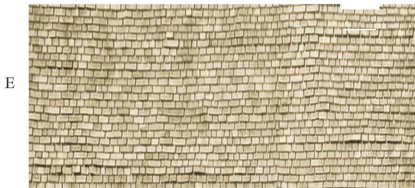
Bottom edge of Front Roof
